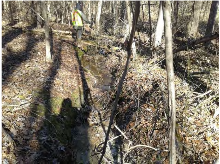
extension S-A18-252 upstream
