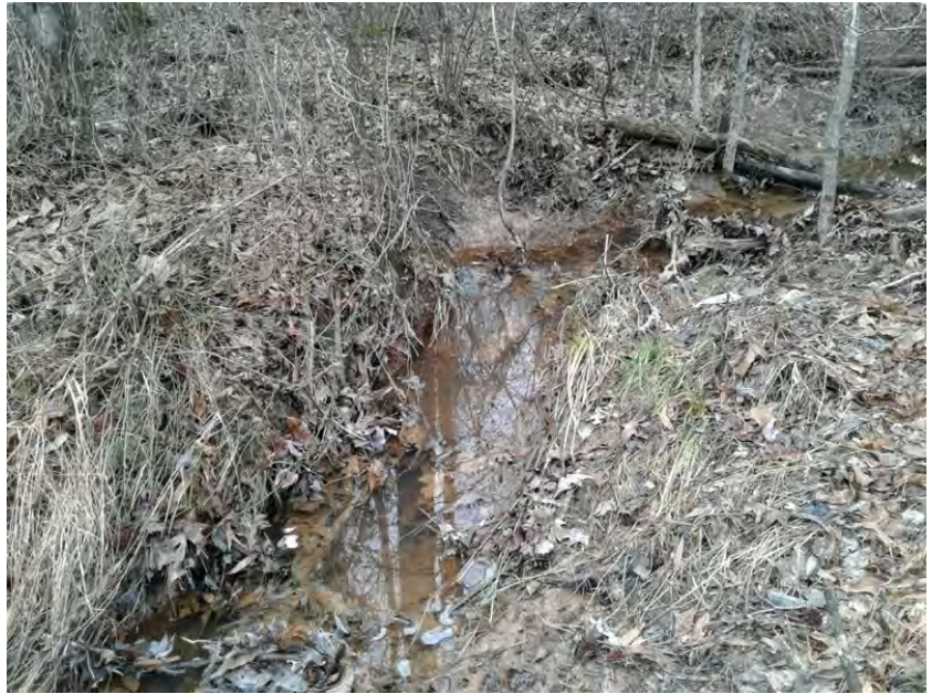
upstream on south side of culvert
