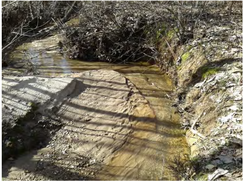
A19 ext-S, downstream, west
