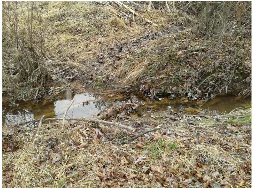
Across stream on south side of culvert, East
