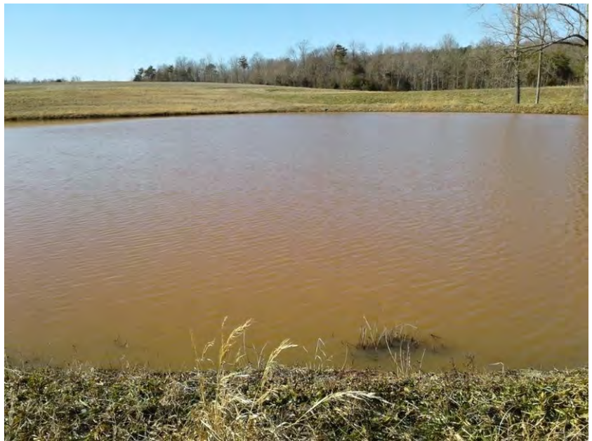
A19 across, north
