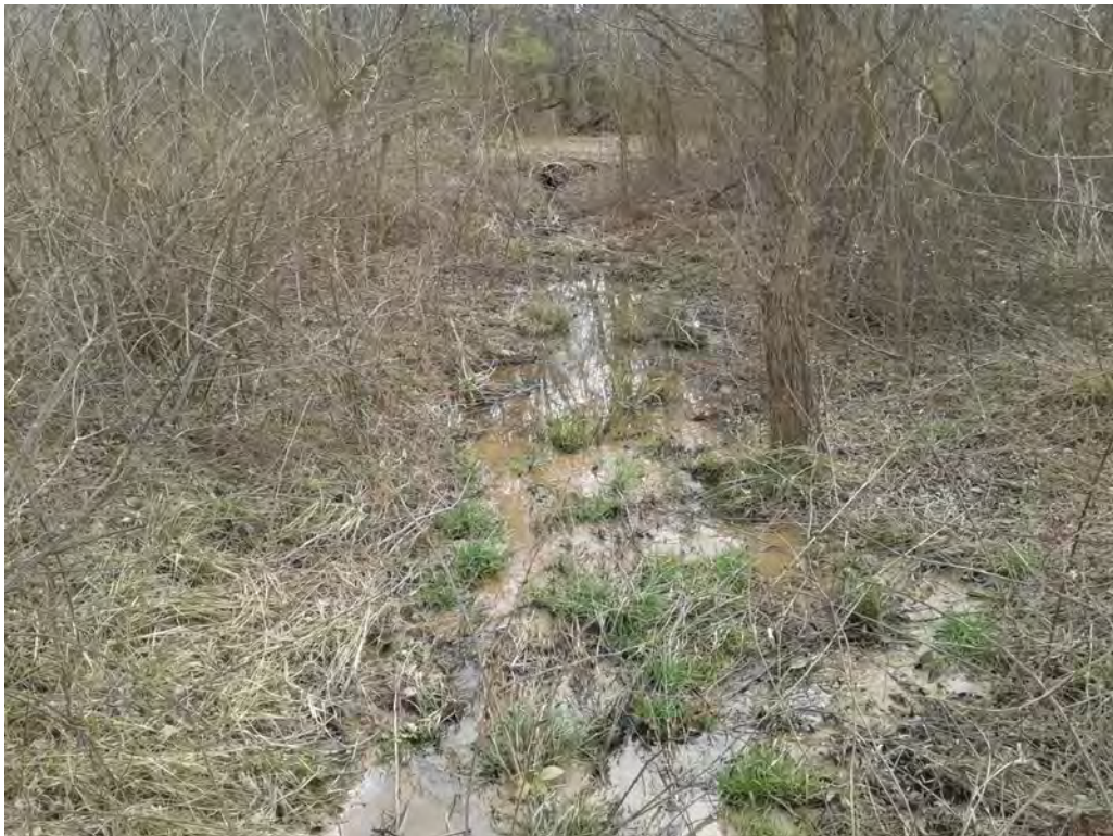
200 series, culvert under road
