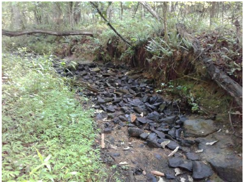
Downstream portion facing upstream
